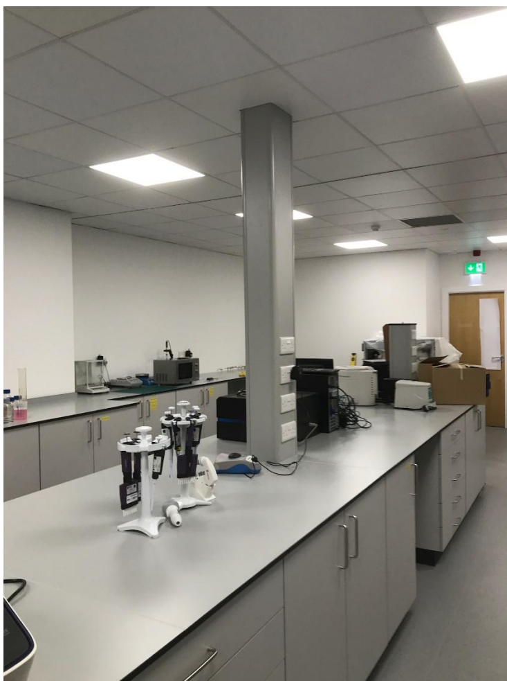
SERVICE DROPPER WITH SOCKET
