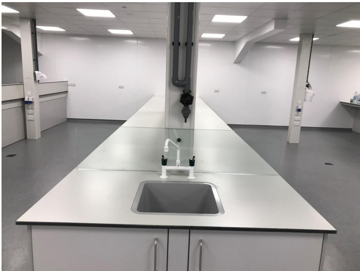
PEDESTAL SYSTEM WITH TRESPA SERVICE DROPPERS
